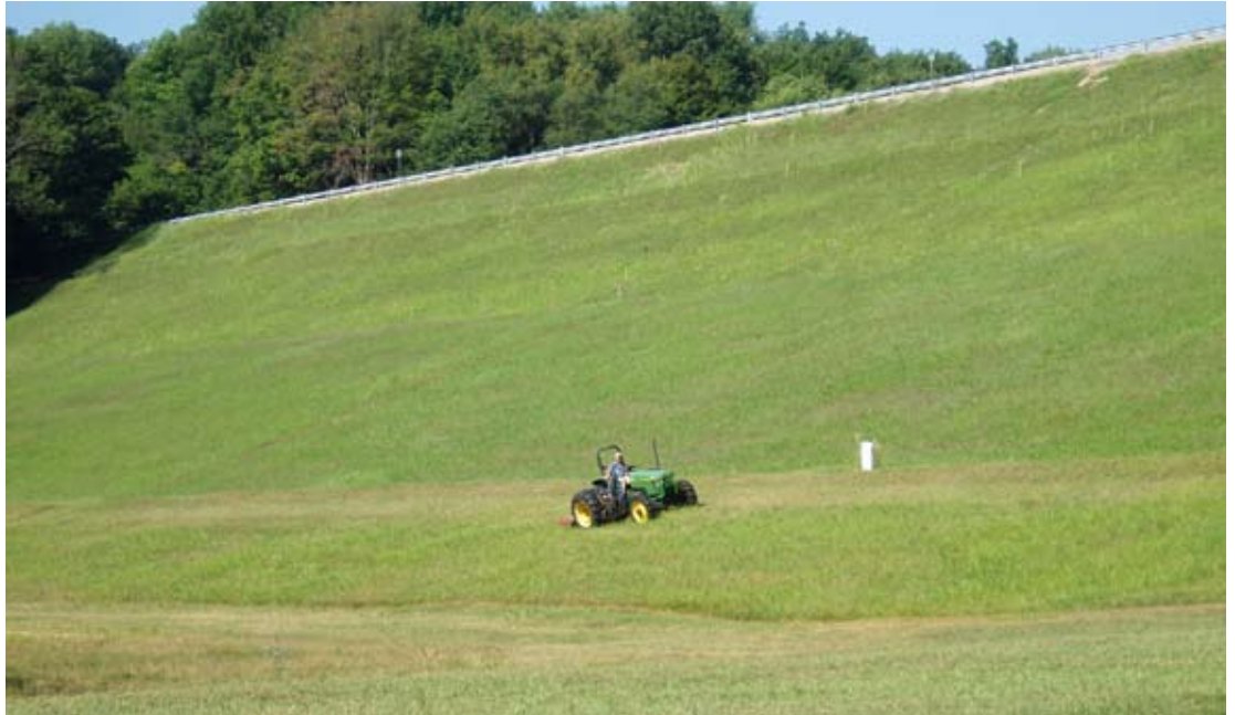
MOWING THE DAMS IS PART OF A COMPREHENSIVE MAINTENANCE PLAN TO ENSURE THE FLOOD PROTECTION SYSTEM WORKS PROPERLY DURING HIGH-WATER EVENTS.
